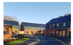
4. Active Homes, Neath, Wales
